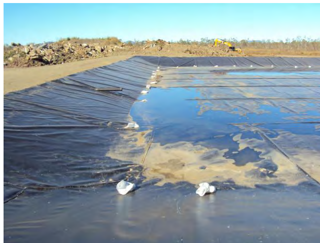
Leachate pond with HDPE liner
