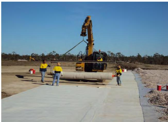
Their work progressed well and Council were satisfied with the high standard of finishing achieved. The Allciv team worked with Council to ensure that the construction made best use of existing site materials and completed the specialist task of the geo composite clay liner and drainage ballast installation in house. It was also pleasing to see the contractors work with the landfill operator to ensure that there was minimal disruption to existing waste disposal operations.
