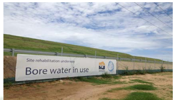
Rehabilitation of a 6.5 hectare section of the Hervey Range Landfill
