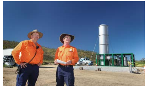
Installation of the second landfill gas flare in Townsville
